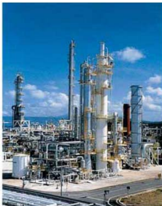
Fig. 3-5: Post-combustion capture at a fertilizer plant in Malaysia [157]
