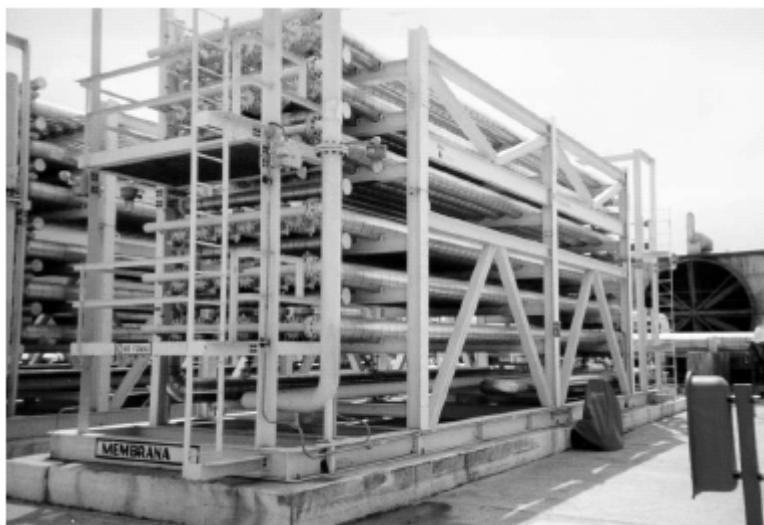
Fig. 3-7: Membrane skid [160]
